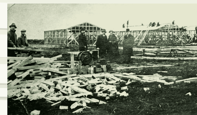
Brocton Camp under construction (Jake Whitehouse)
