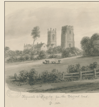
A 1843 drawing by John Buckler entitled Approach to Rugeley from the Stafford Road. The picture shows the towers of both the current St Augustine's church and the original parish church that it replaced. Courtesy of the Trustees of the William Salt Library, Stafford
