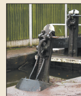
Sturdy paddle-gears are used to control the flow of water in and out of locks.
