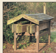
These planks kept in a shelter are used to seal a lock when maintenance work is done. They slot into the notches you can find on canal bank stonework.
