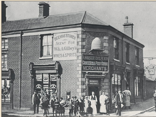
The Beehive Stores, c1900. Many local people remember the distinctive 'beehive' that was fixed to the wall above the doorway, but no-one knows what happened to it when the shop was demolished. Image courtesy of the Museum of Cannock Chase
