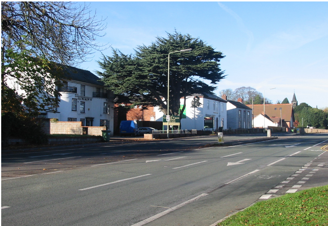
Fig. 4 Potential area for enhancement using less visually obtrusive traffic management on Main Road.
