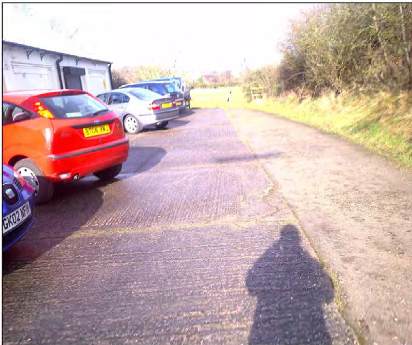
Photograph 6: Coach and general car parking area in the central portion of the site. Hardstanding appears to be in a good state of repair and no oil / fuel staining was noted during the walkover.
