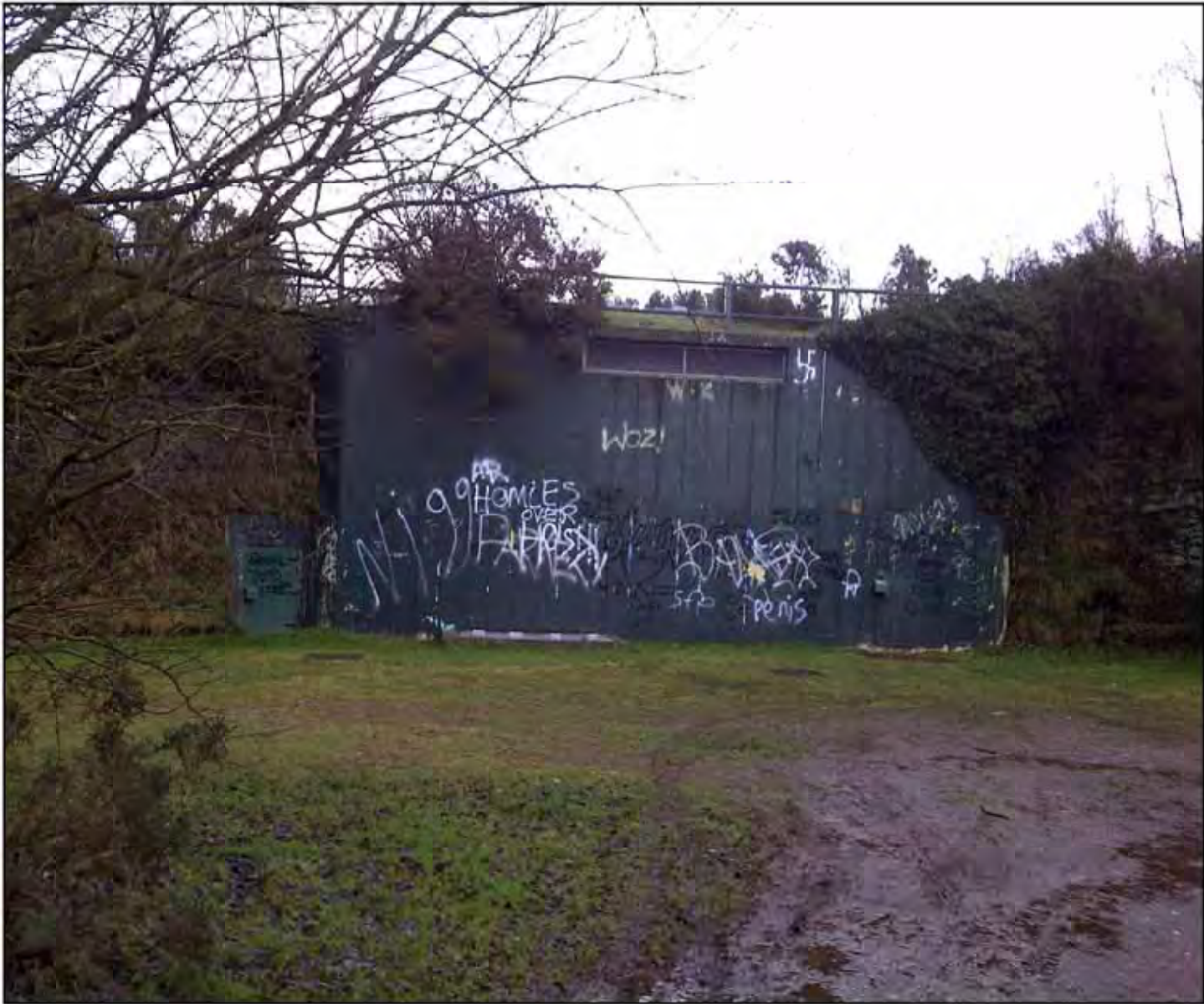
Photograph 5: Unknown plant storage / mining shaft entry point. The feature is securely locked and is no longer in use.
