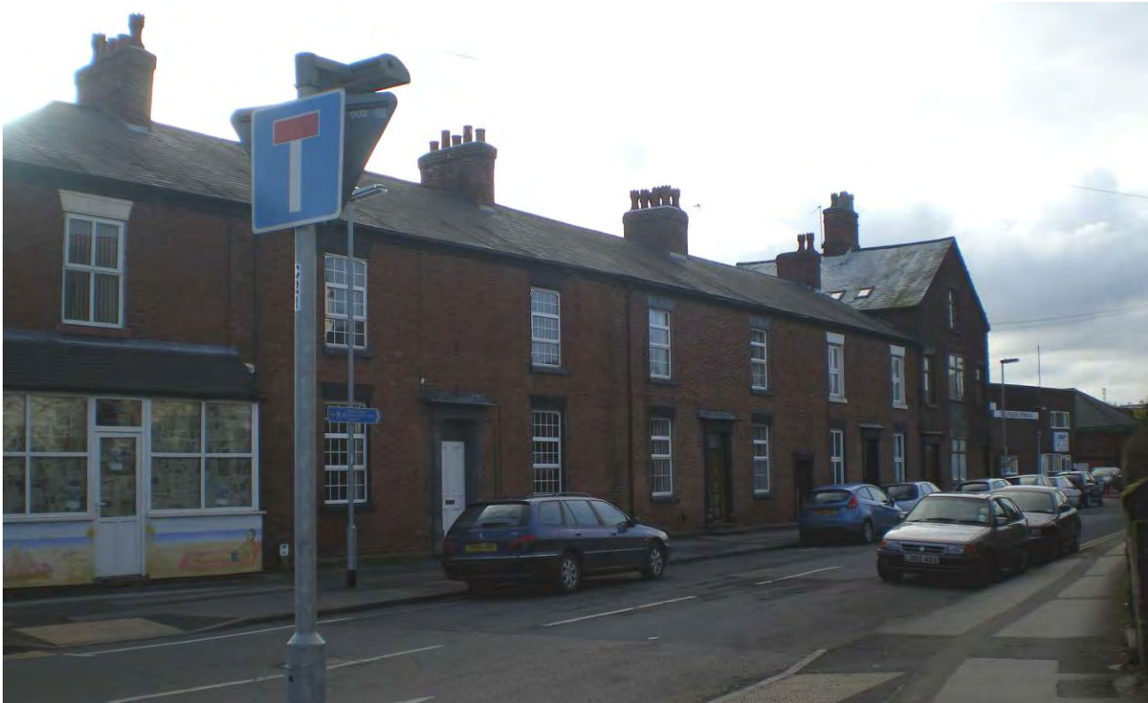
Plate 12: 19th century properties in Market Street
