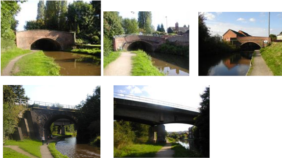
Fig. 10 (upper row from left) Bridge 64, 65, 66;(lower row from left) Listed railway Viaduct and disused concrete bridge
