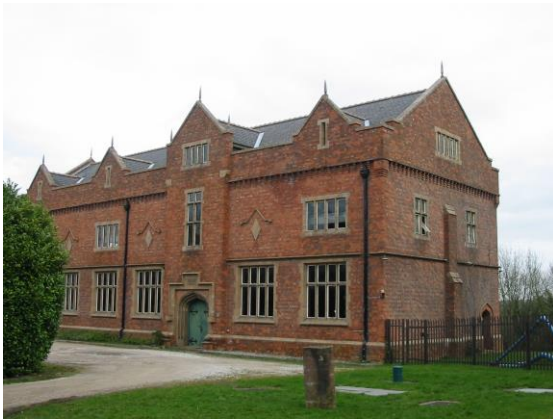
Fig. 1 Brindley Bank Pumping Station
