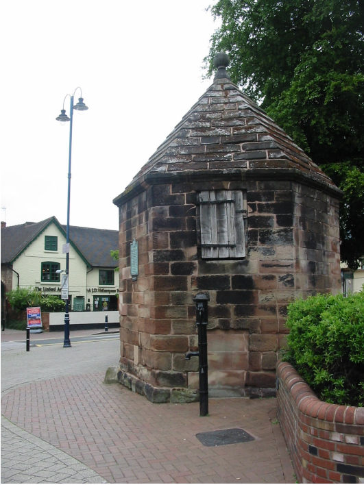
Fig.5 : Conduit building and water pump
