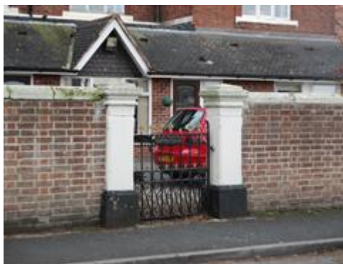
Fig. 8 Front wall, gateposts and gate at 30 Church Street
