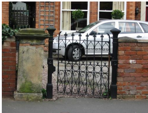
Fig. 9 Wrought iron gate and gate piers at 8 Church Street
