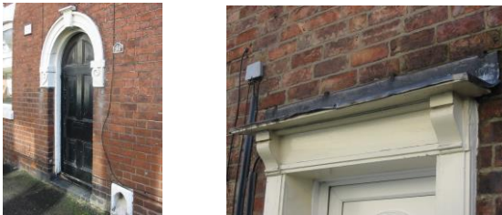
Fig 5 Panelled door and doorcases in Bow Street
