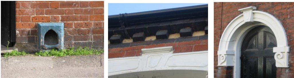
Fig. 7 Bootscraper, dentilled eaves and door head in Bow Street
