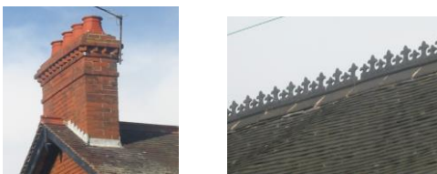
Fig. 6 Decorative chimney and roof in Sheepfair
