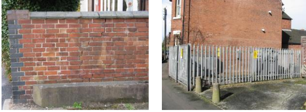
Fig.4 Old boundary wall in Taylors Lane and sub-station fencing in Sheepfair
