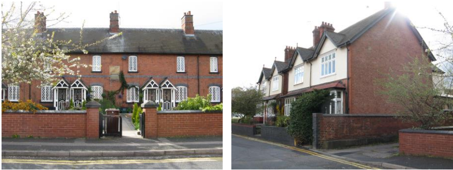
Fig. 2 Almshouses and villas in Taylors Lane
