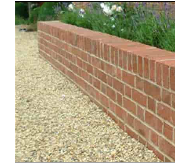
Brick dwarf wall
