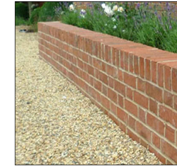
Brick dwarf wall
