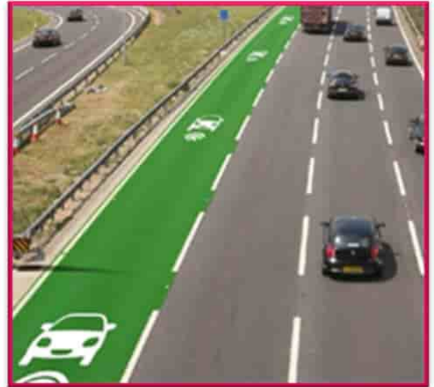
Figure 39: Wireless in road charging
