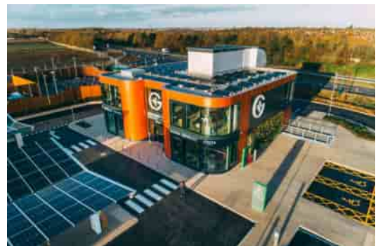
Figure 38: GRIDVOLT charging hub
