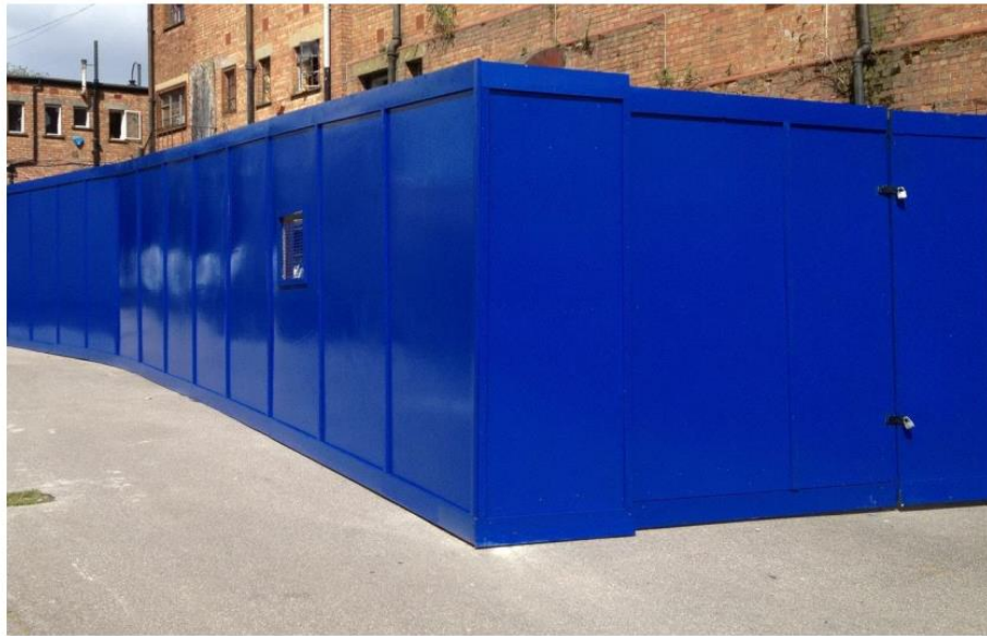
Figure 8: Extract from Demolition Method Statement showing the type of hoardings to be erected around the site
