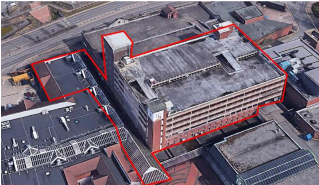
Figure 1: Extract from submitted Demolition Method Statement depicting the extent of the zone of demolition proposed. Members attention is drawn to the excluded area above Home Bargains and Peacocks which other than removal of the lift shaft element, will remain.
