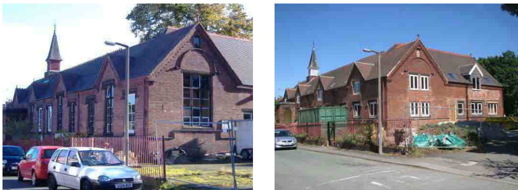
Fig. 4 The former Talbot Street School, before and during conversion to residential use.
