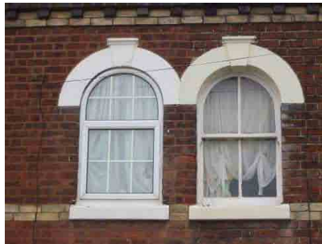
Fig. 12 comparison of original and replacement windows
