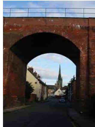
Fig. 6 View through Arch Street bridge
