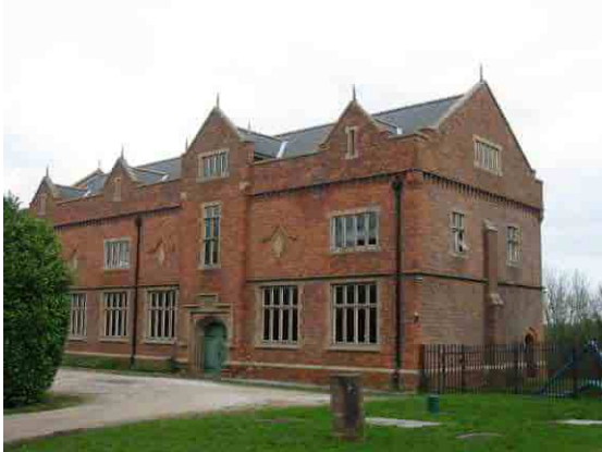
Fig. 1 Brindley Bank Pumping Station
