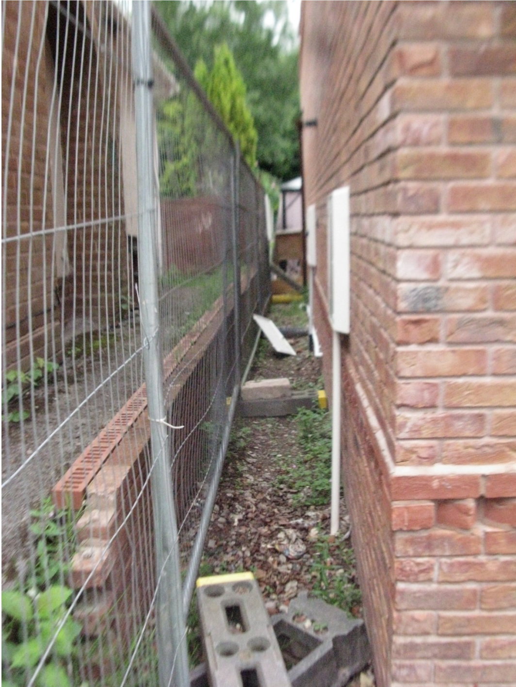
Photograph Showing the Relationship Between the Sider Elevations of the Dwelling AS-Built and No66 New Penkridge Road
