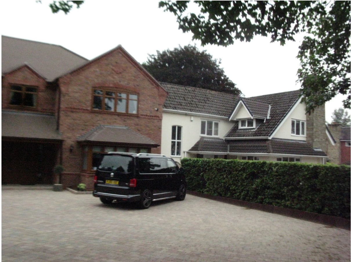
Photograph showing the Relationship between the Dwelling As-Built and the Neighbour at No 62c New Penkridge Road
