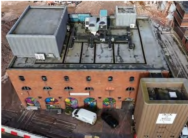
Fig 5 - Aerial view of the respective flat roof areas.
