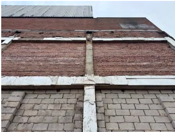
Fig 19 - View of exposed south elevation where adjoining buildings have been removed.
