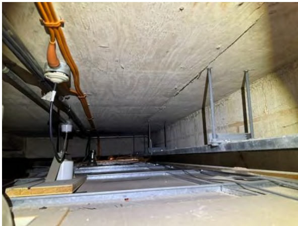
Fig 9 - View of cast in situ concrete floor soffit (second floor).
