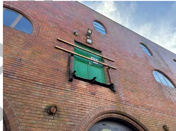
Fig 20 - View of west elevation where link bridges / means of escape have been removed.
