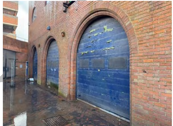
Fig 24 - View of loading doors to the former market hall areas.
