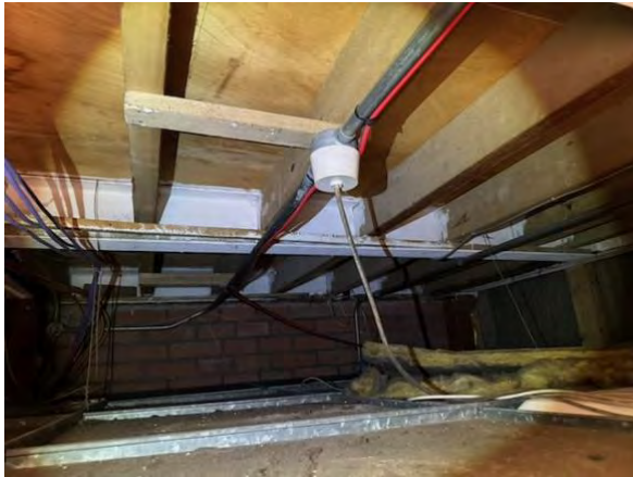
Fig 25 - View of limited suspended timber flooring to link bridge and landing areas.
