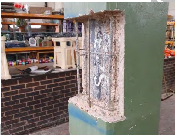
Fig 13 - View of previous investigations showing the steel frame, concrete encasement and steel reinforcement
