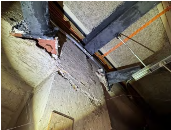
Fig 3 - View of concrete encasement to steel column and beams, including exposed steel bracing
