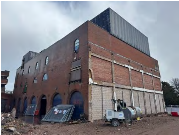
Fig 7 - View of the south and west elevations, including the cladding to the stage fly tower.
