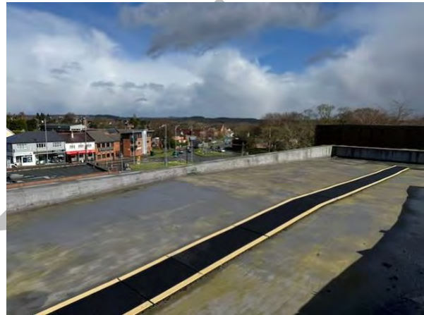
Fig 6 - View of the principal flat roof which falls to the east and west elevations.
