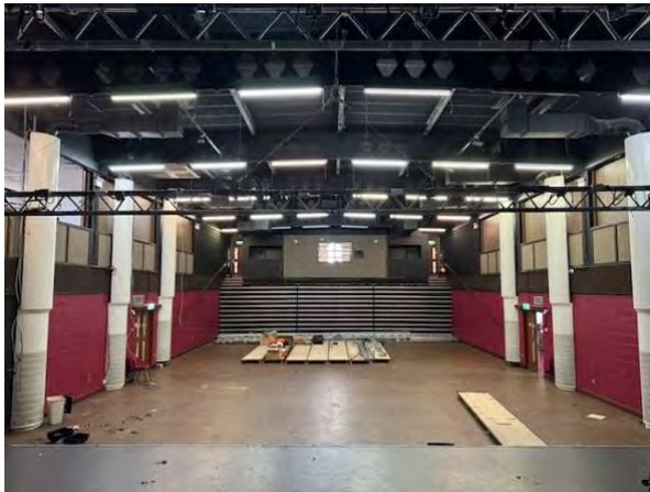
Fig 11 - View of the auditorium and retractable seating.
