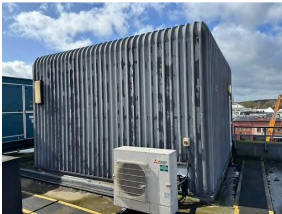
Fig 21 - View of the profiled metal cladding to the north west stairwell.
