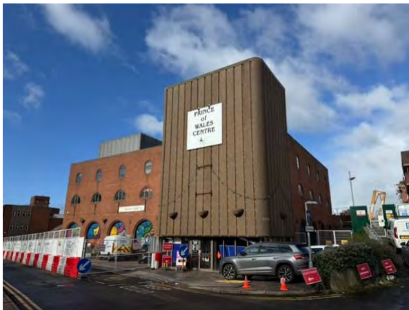
Fig 1 - View of front (east) elevation and main entrance to the property.
