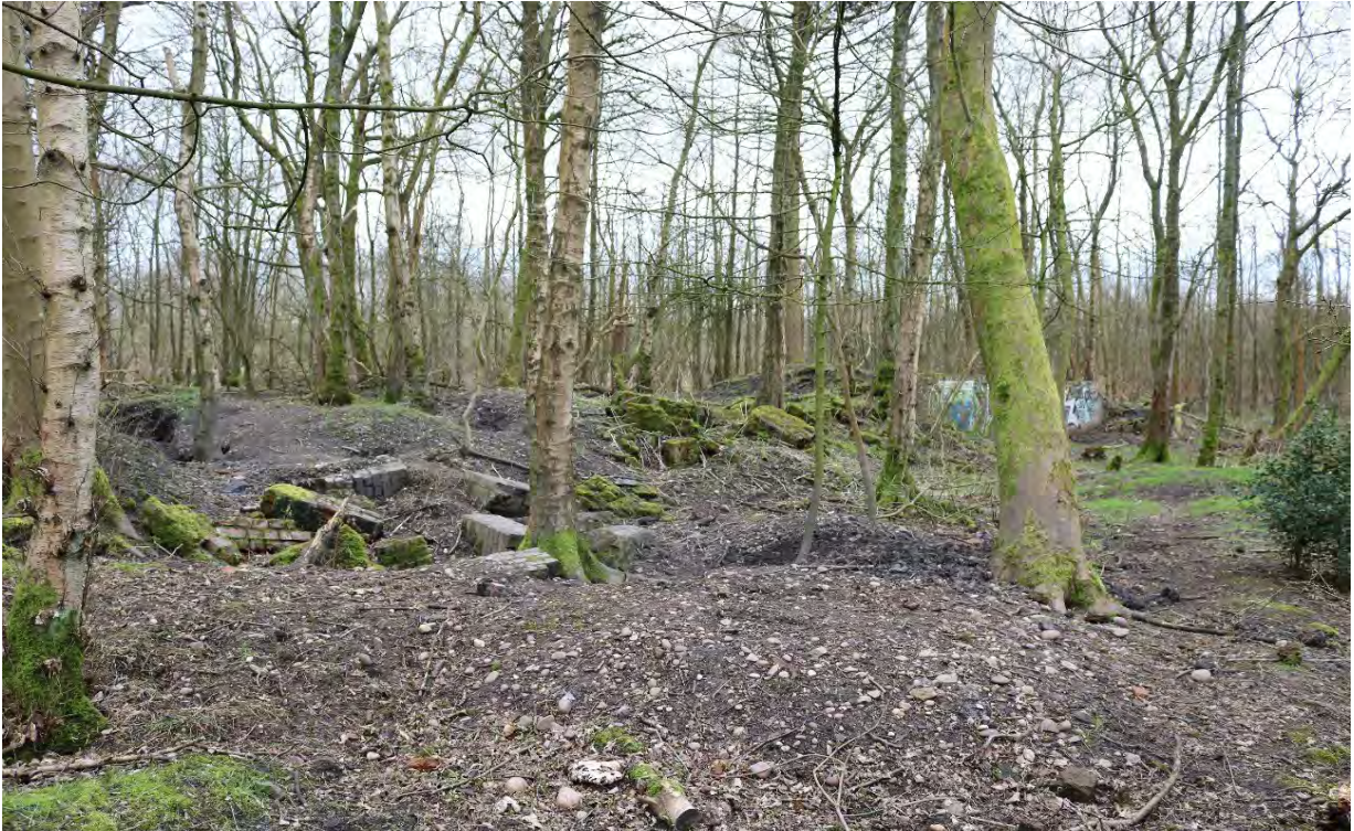
Image EDP A1.3: View illustrating the demolition rubble of the Cannock Chase Colliery in the north-east of the Site. View looks east across rubble in the eastern part of the former colliery.
