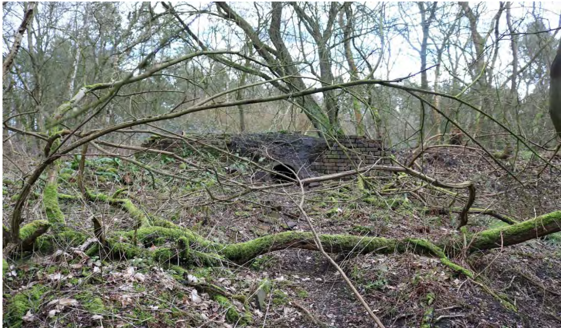
Image EDP A1.2: View illustrating the limited remains of the Cannock Chase Colliery in the north-east of the Site. View looks east toward a pipe and masonry on the western edge of the former colliery.
