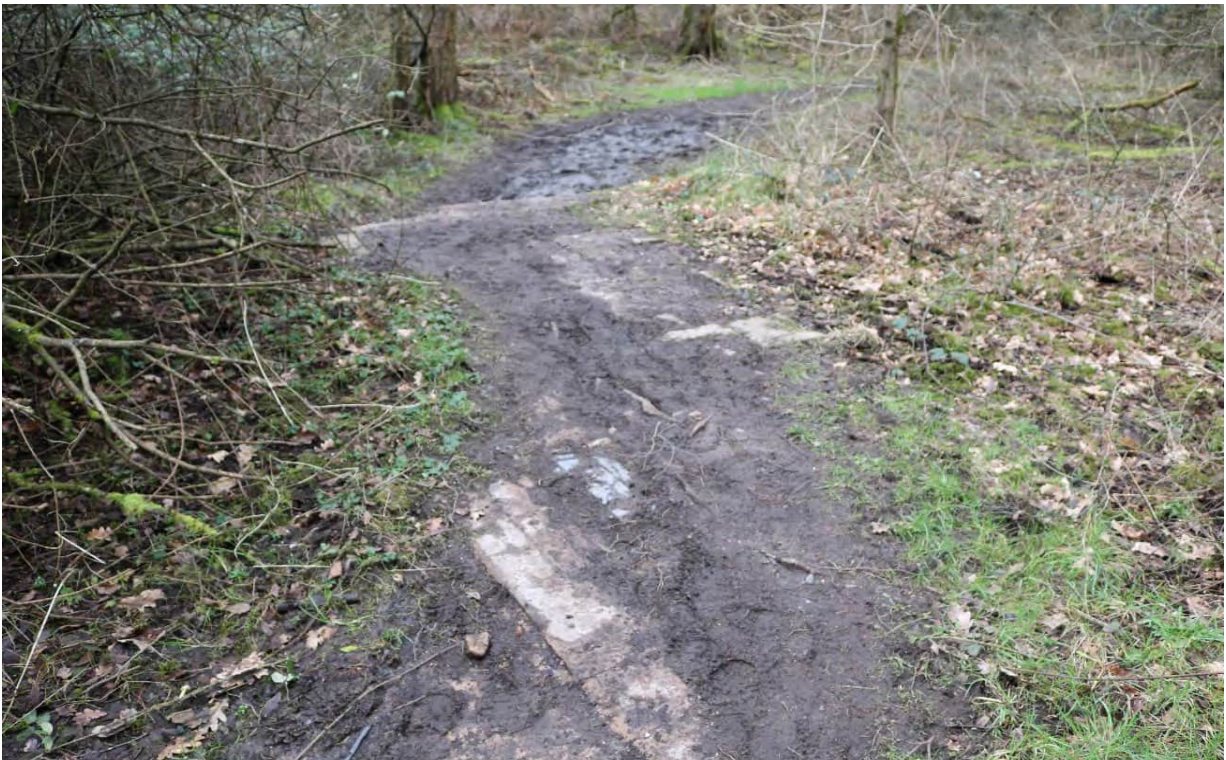
Image EDP A1.4: View illustrating the extent of the demolition of Cannock Chase Colliery in the north-east of the Site. View looks north-west across apparent remains of floor and walls in the north of the former colliery area.
