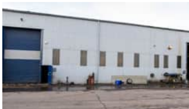
Existing industrial unit - Watling Street site
