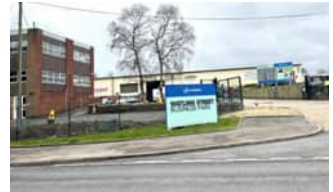
Existing entrance- Watling Street site
