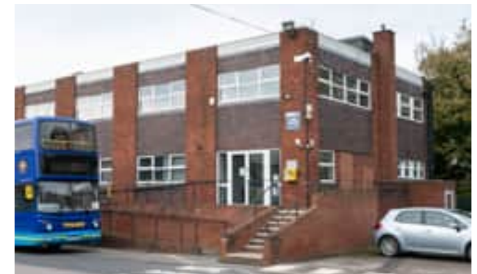
Existing office building (Oak House) - Watling Street site
