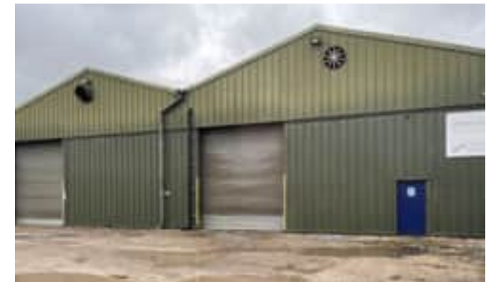
Existing industrial unit - Watling Street site
