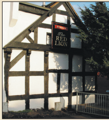
The Red Lion, which is the oldest licensed premises in the town, is a timber-framed building dating from about 1600. This type of timber-frame is called a box frame.
