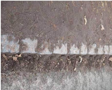
Granite setts used in kerbing
