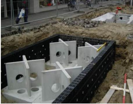
Root box constructed under paving
