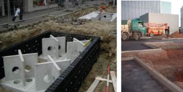
Root box constructed under paving
