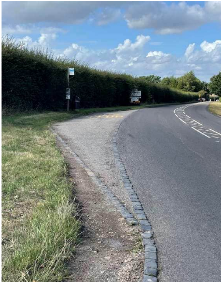
Figure 8: Bus Layby, Westbound - Haughton, Staffordshire
