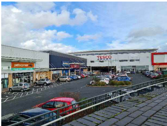
Photograph 4: Victoria Shopping Park
