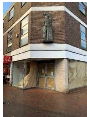
Photograph 7: Vacant unit at the corner of Bees Lane and Lower Brook Street
