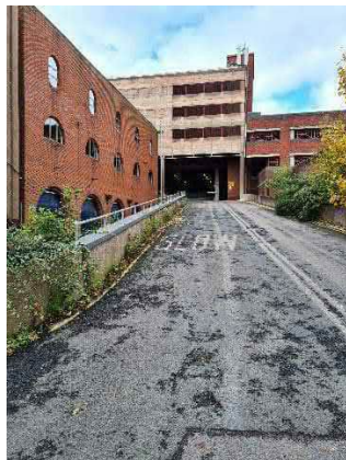
Photograph 7: Ramp to the closed multi-storey car park
